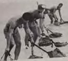
THE CHARGES were in inflatable cases to facilitate movement in the water when the men reached the site they punctured the bags, letting the charges settle on the ocean floor.
