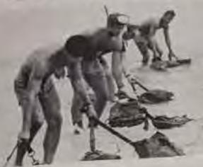
THE CHARGES were in inflatable cases to facilitate movement in the water when the men reached the site they punctured the bags, letting the charges settle on the ocean floor.
